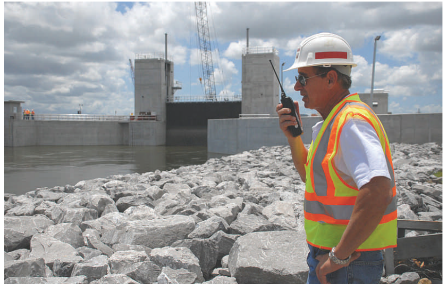
Chris Accardo, Chief, Operations Division, oversees activities at the Seabrook Floodgate Complex on Media Day. USACE Photos by Paul Floro
